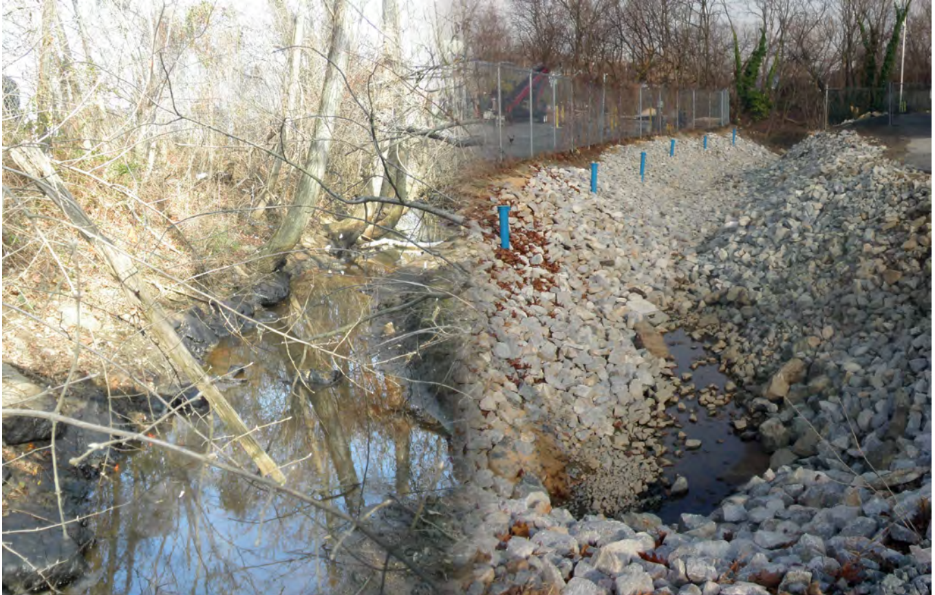
View of the Mecco Drive Ditch Before and After Remedial Activities
